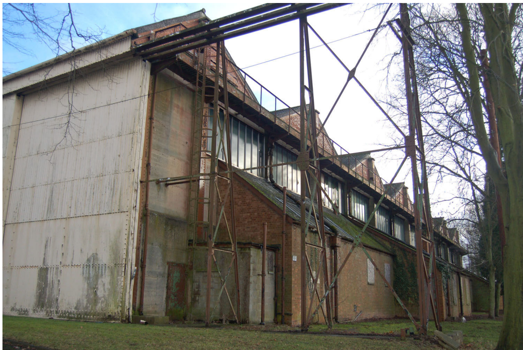
Building 79 A type hangar
